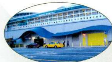
An existing warehouse was transformed over eight weeks into a passenger check-in facility.
